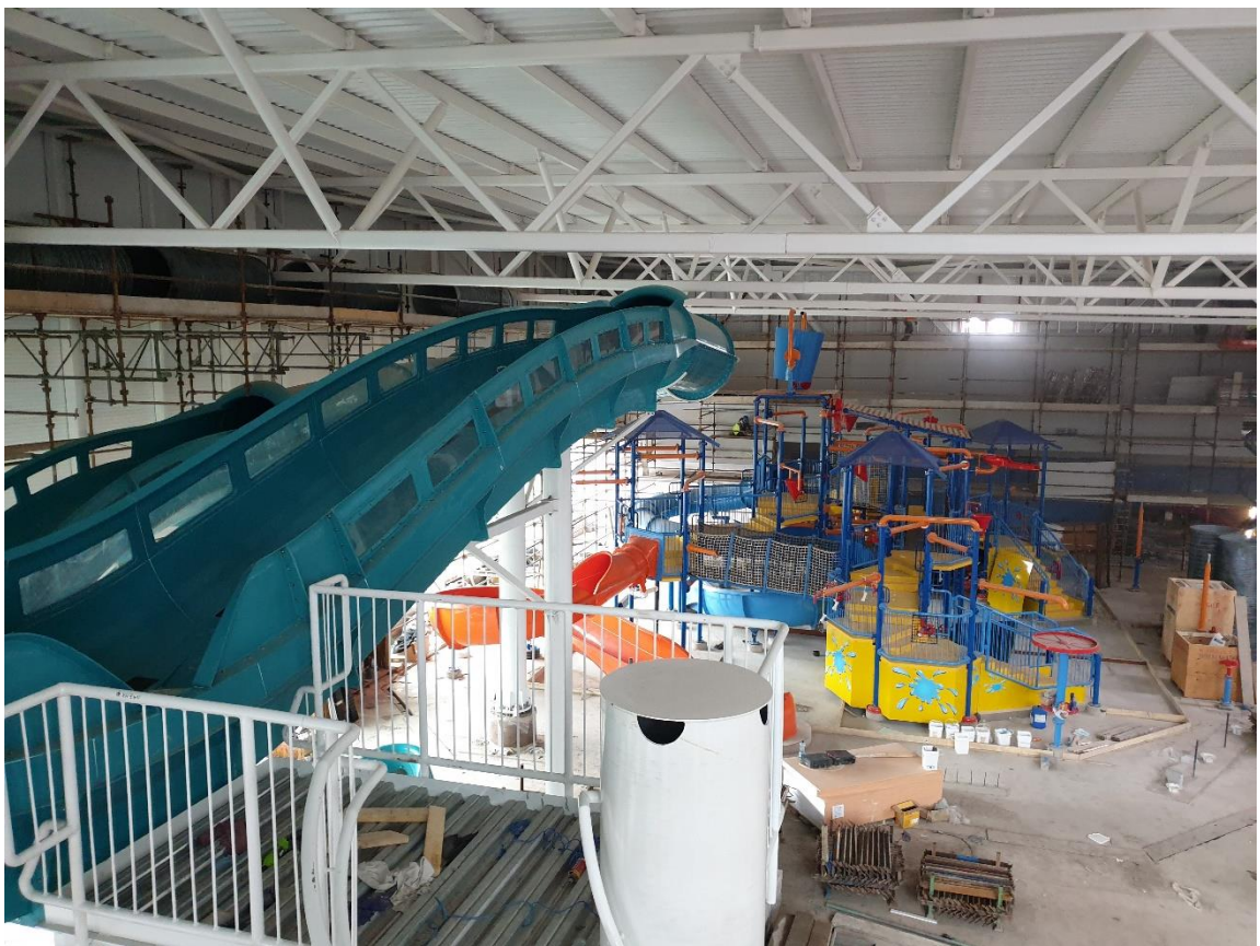
Andersonstown- main pool hall
